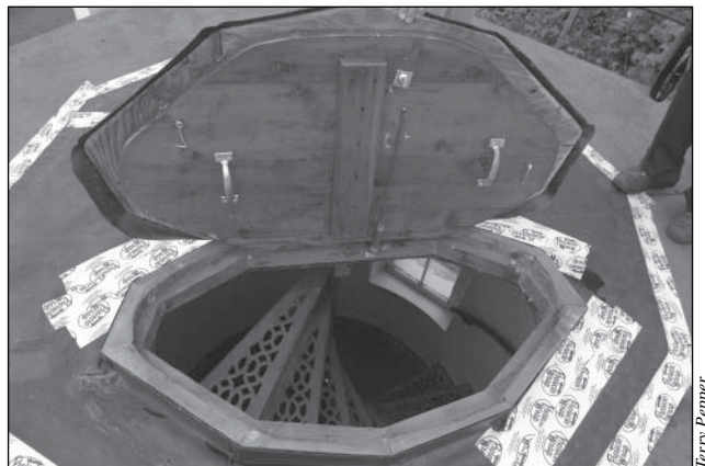
The original cast iron scuttle door was likely removed at the same time as the lantern, and has been replaced by this wooden door
