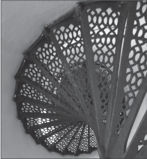
These intricate cast iron spiral stairs within the tower still serve as the only means of access between the floors in the dwelling
